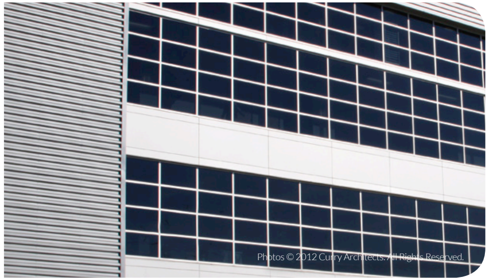
Mustang Stadium includes a turf field for football, field hockey, lacrosse and soccer. The signature element of the building is the exterior brick, metal and glass façade that was fabricated with approximately 2,700 square feet of Solarban ® R100/ Solargray ® glass by Vitro.
